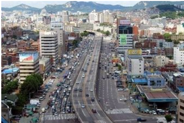
June 2003 Before Restoration ♪
