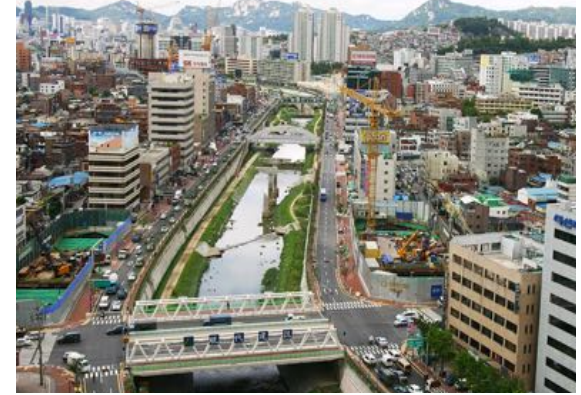
September 2005 After Restoration ♪
